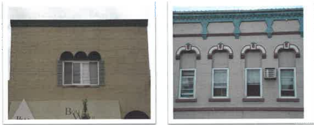
Figure 2.13: Discouraged Windows – Windows that are both not to scale with the façade or the traditional window openings.
