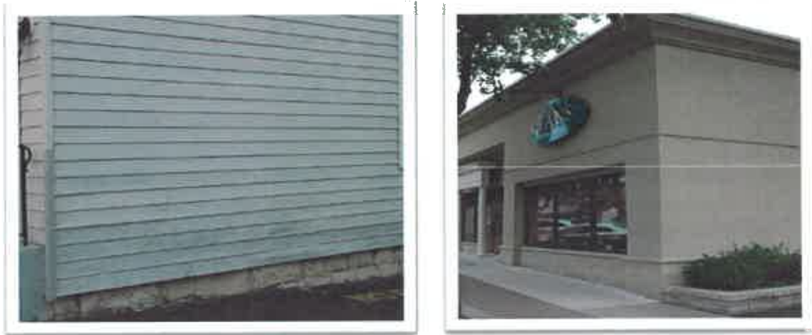
Figure 2.07 Discouraged Materials: Discouraged – vinyl and aluminum siding, and EIFS as a primary material.
