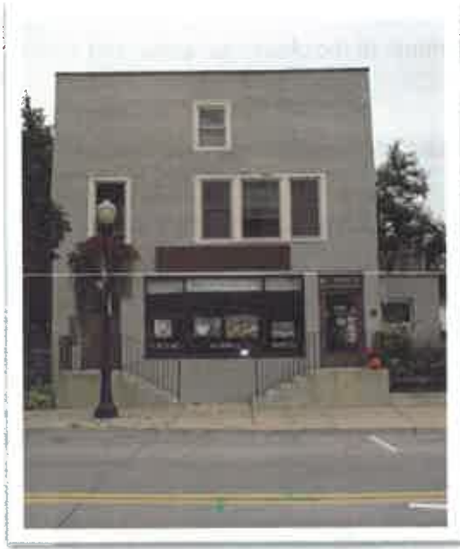
Figure 2.10 Discouraged Façade: These figures illustrate poor design through lack of detail, poorly spaced windows and doors, no sense of top, middle, and base, and minimal variation in materials and brick color.
