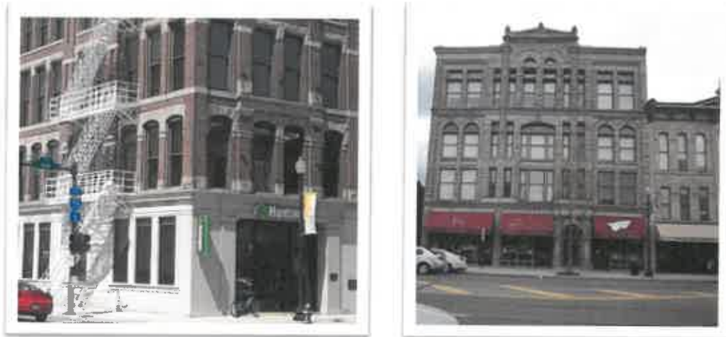
Figure 2.06 Appropriate Building Materials: Good use of brick, stone, and canvas awnings.
