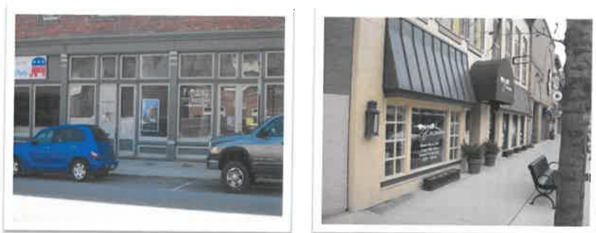
Figure 2.16: Encouraged Storefront – Knee walls and windows making up the majority of the storefront demonstrate a strong base.
