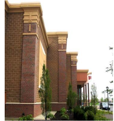
Figure 1161.2 - 2 Vertical Articulation – Recess
