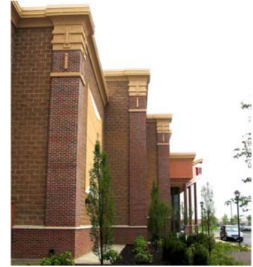
Figure 1161.2 - 2 Vertical Articulation – Recess
