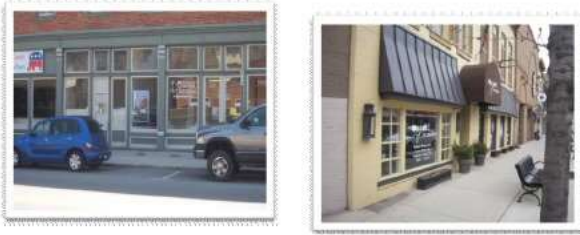
Figure 2.16: Encouraged Storefront- Knee walls and windows making up the majority of the storefront demonstrate a strong base.
