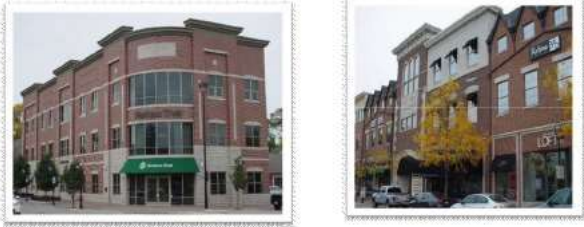
Figure 2.09: Encouraged Building Façade - These figures exemplify use of similar and complementary materials, proportionate well-spaced windows, appealing building details, and well-defined top, middle, and base.
