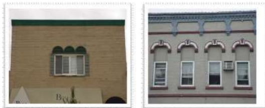
Figure 2.13: Discouraged Windows- Windows that are both not to scale with the façade or the traditional window openings.
