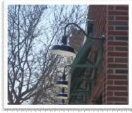
Figure 2.25: Encouraged Projecting lights - Projecting lights
