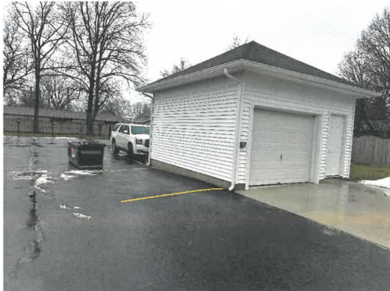
Striping on Lot to Create (1) Additional Parking Space
