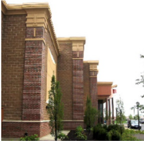
Figure 1161.2 - 2 Vertical Articulation - Recess
