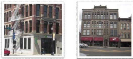
Figure 2.06 Appropriate Building Materials: Good use of brick, stone, and canvas awnings.
