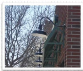
Figure 2.25: Encouraged Projecting lights - Projecting lights
