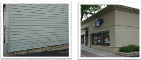
Figure 2.07 Discouraged Materials: Discouraged - vinyl and aluminum siding, and EIFS as a primary material.
