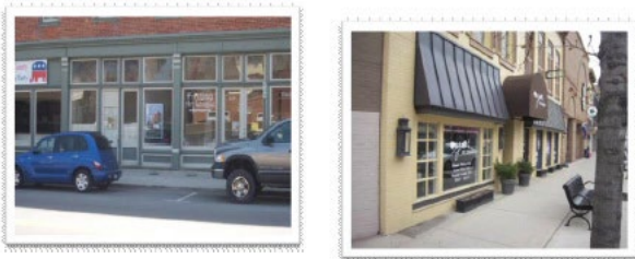
Figure 2.16: Encouraged Storefront- Knee walls and windows making up the majority of the storefront demonstrate a strong base.
