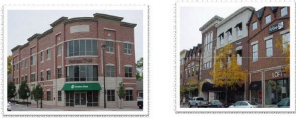
Figure 2.09: Encouraged Building Façade - These figures exemplify use of similar and complementary materials, proportionate well-spaced windows, appealing building details, and well-defined top, middle, and base.
