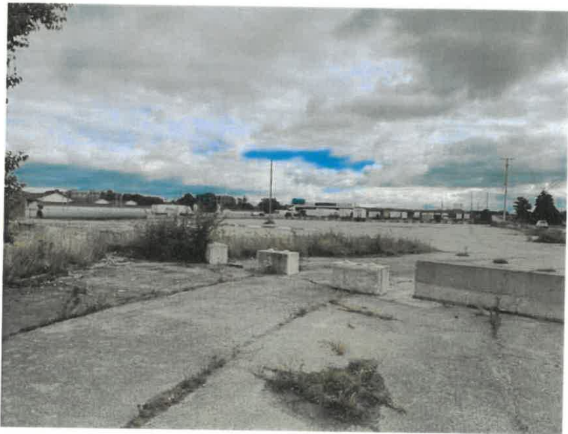
View of 325 Emma Street looking south
